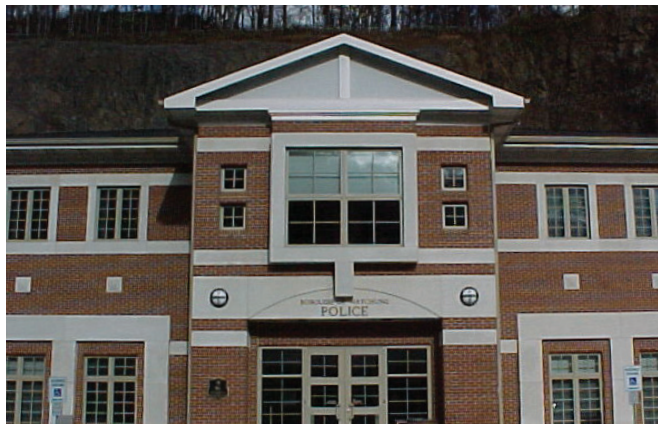
Watchung Police & Court Facilities, Watchung 2002 Recipient
