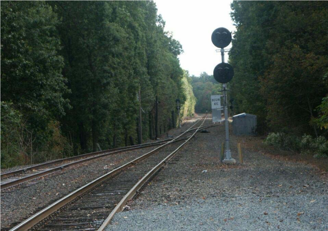
Abandoned Tracks North of High Bridge Station – Raritan Valley Line
